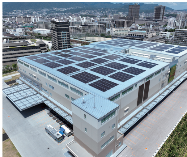
Solar panels installed at the Hanshin ALC* of MEDICEO CORPORATION
