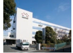
KANAGAWA ALC (first ALC)
