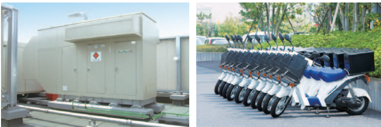
In-house power generator and emergency shipping motorcycles for use in the event of a disaster
