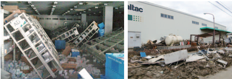
Damage from the earthquake and tsunami: Spilled inventory at MEDICEO CORPORATION's Sendai building warehouse (left) and Paltac Corporation's RDC Sendai (right)
